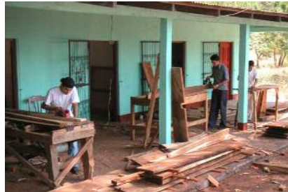
The carpentry workshop in SFL
