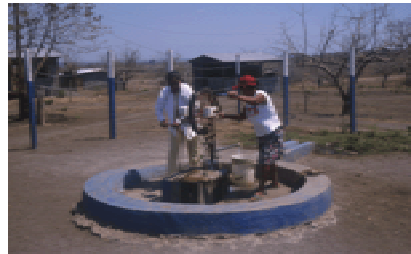
Pump in Santa Rosa
